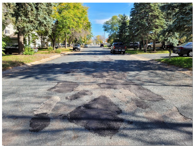
Exhibit 5. Norton Avenue looking east.
