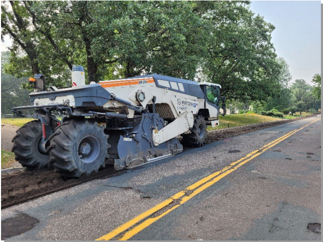
Exhibit 1. Full-depth pavement reclamation.
