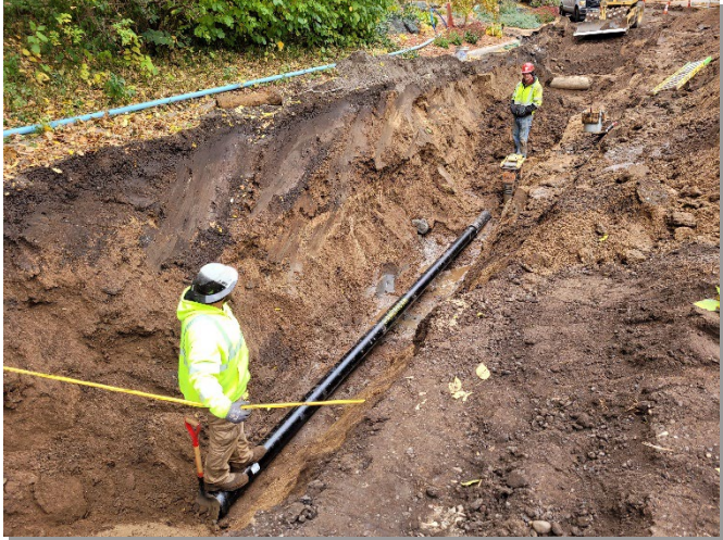
Exhibit 7. Water main replacement.
