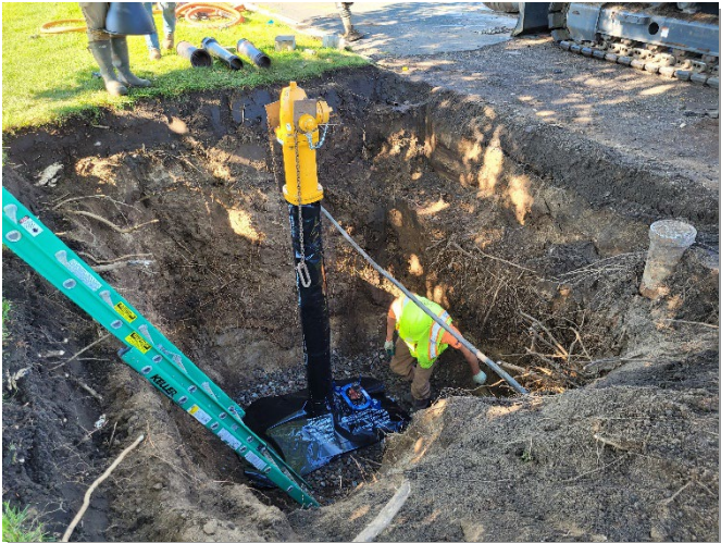
Exhibit 8. Fire hydrant assembly replacement.
